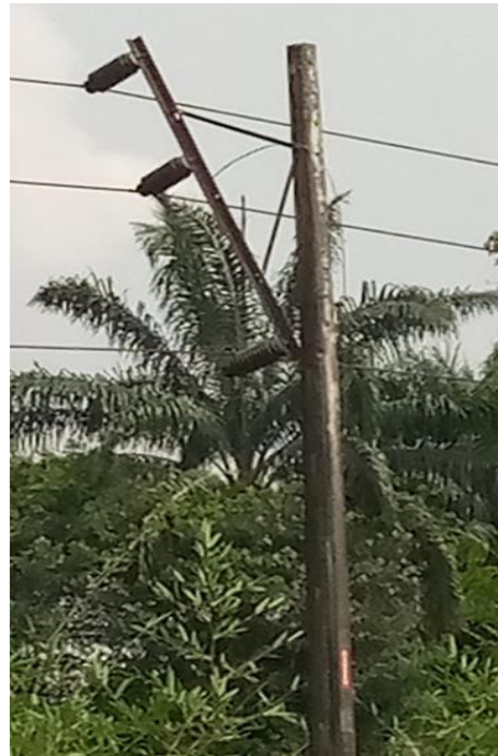
Figure 2: Insulator attached directly to the utility pole at Oleh Community. Figure 3: Hanging cross arm at Emede Community.
