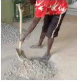
Figure 2: Dry mix of aggregates
