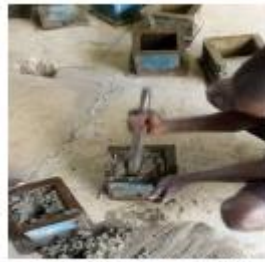
Figure 3: Concrete cubes casting
